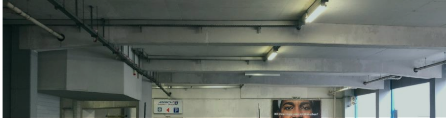
Existing beams in parking space
